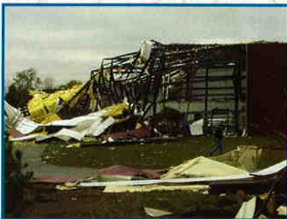
Following an F3 tornado, Busk Brothers' precast building, utilizing Fabcon's VersaCore™ panels, sustained only minor cosmetic damage. Adjacent buildings, such as the one on the left, were severely damaged or destroyed.
